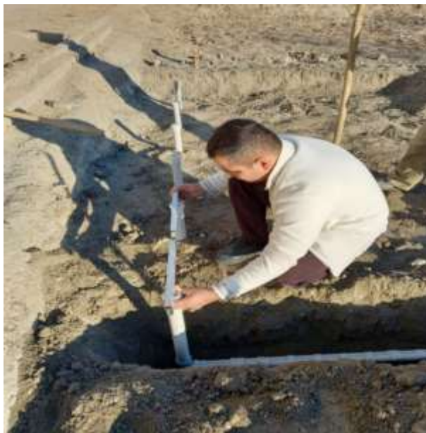
1-Figure . Installation of plastic pipes under the soil on the experimental plot.
