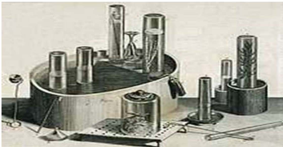
6-rasm. Pristlining gazlarni simob ustida yig‘ish asbobi.
