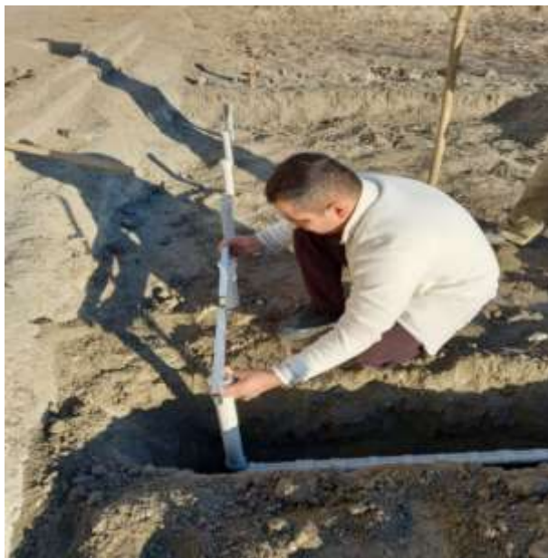
1-Figure . Installation of plastic pipes under the soil on the experimental plot.
