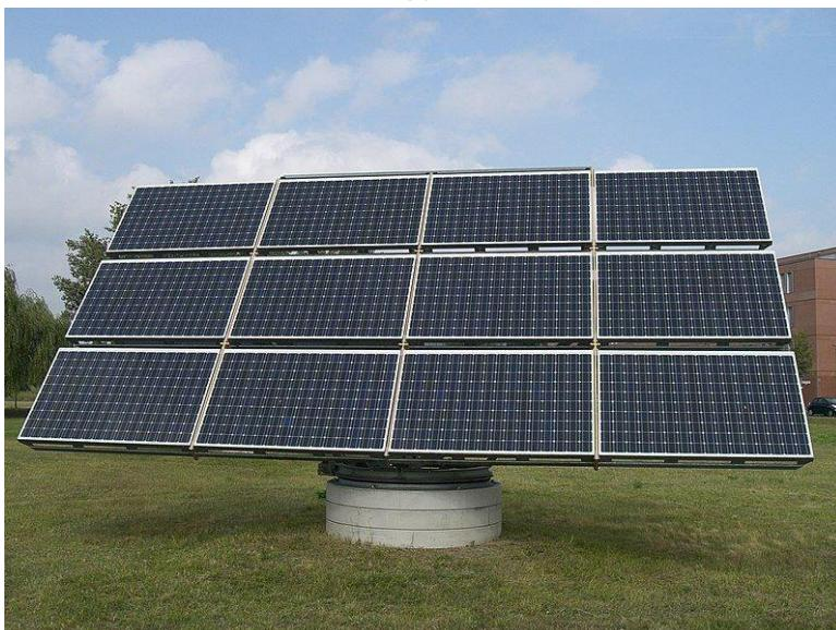
The best thing about the two-axis solar observing equipment is that they travel along the solar trajectory during the day on the azimuth and Zenith axis, ensuring that sunlight falls perpendicular to the surface of the solar photoelectric panels. The initial investment costs required for two-axis solar tracking equipment can justify itself in the short term.
