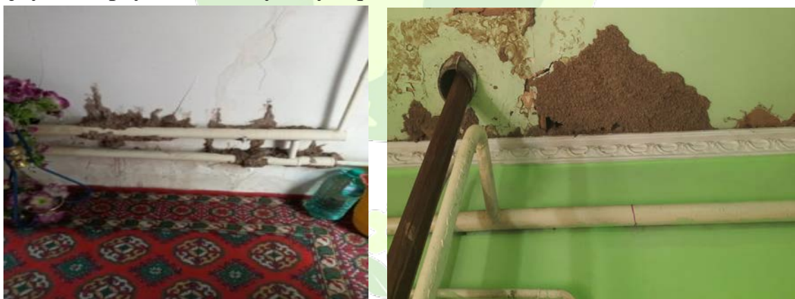
1-rasm. Eski uylarda isitish trubalari yaqinda termitlarning to`planishi.
